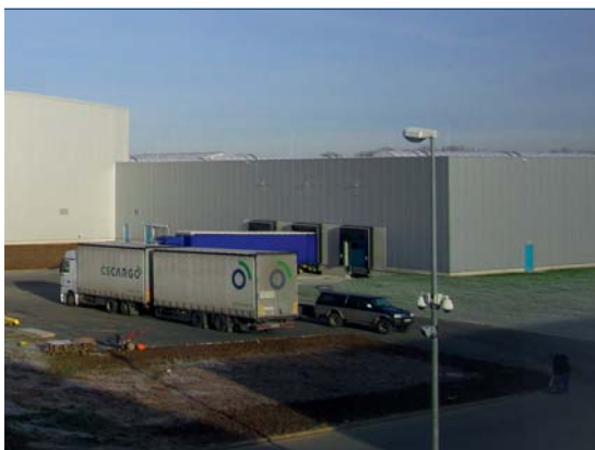
The new hall at WESTFALIA acts as a storage area for coils, tools and finished parts.
